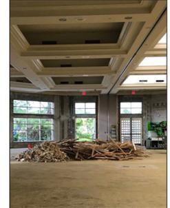
Even the Wood Studs in the Ballroom Had to Be Removed Due to Water Damage
